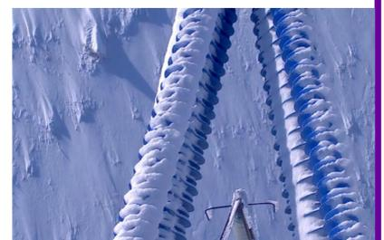
Figure 3 - Composite cross-arm top view recorded on 01 December 2010
